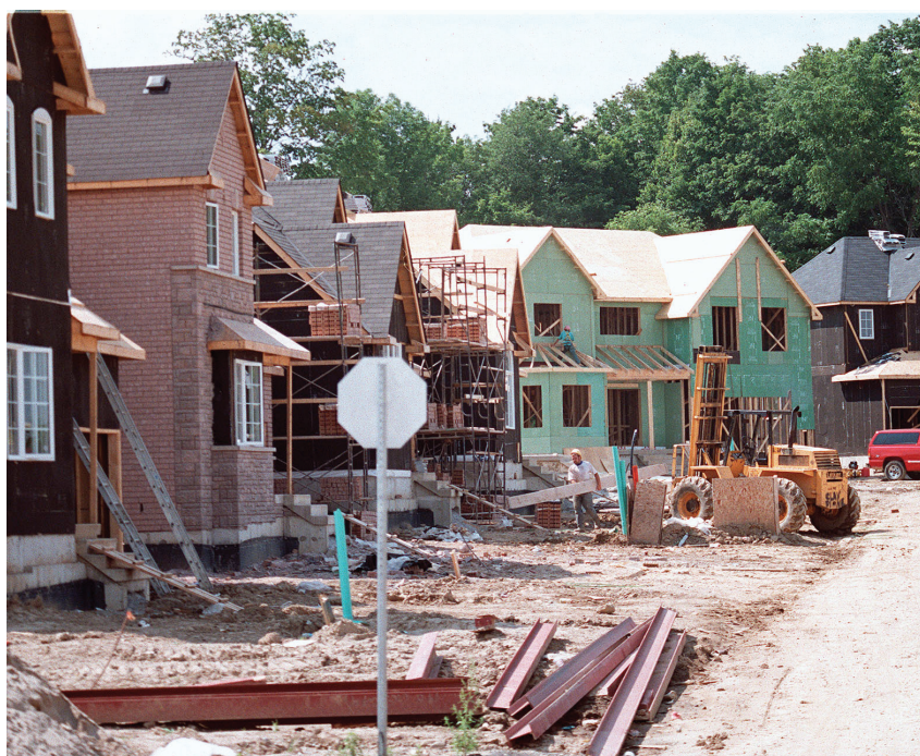
Homes built since 2017 use 15% less energy than homes built just five years earlier. Toronto Star, Brian Dexter / Contributor
